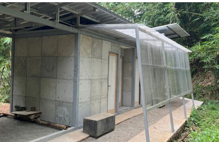
WORLD'S FIRST HOUSE MADE WITH NAPPY-BLENDED CONCRETE - MUHAMMAD ARIEF IRFAN
