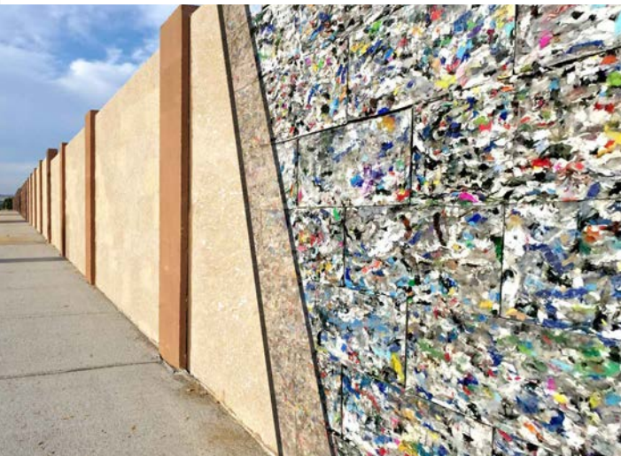
BYBLOCK STUCCO BOUNDARY WALL
