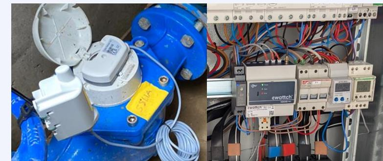
Meters communicating water and electricity readings
