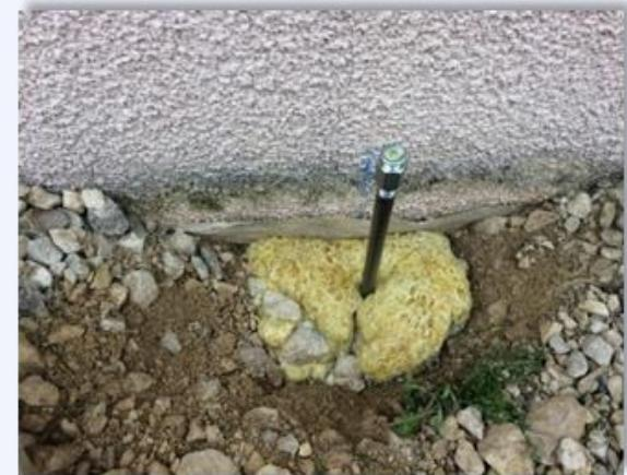
*\*In the particular case of clay soils, which are subject to shrinking/swelling, resin may only be used if certain criteria are met with respect to the plasticity index (PI) and methylene blue (MB) stain test, as indicated in the G5 geotechnical study.*
