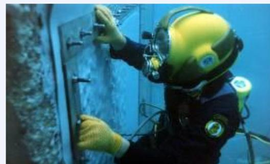
*A SIBELON® geomembrane being rolled out, positioned and fixed in place underwater*
